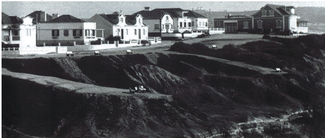
Fig. 3.2.4 The first buildings along the coast of Praia da Areia Branca
