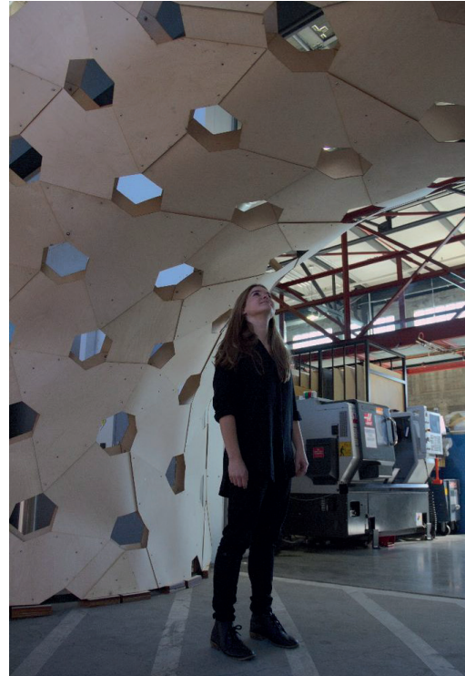
Fig.2.4.4 Bending-Active structure, developed by ITKE engineer and researcher Riccardo La Magna during the residency period at Autodesk's Pier 9
