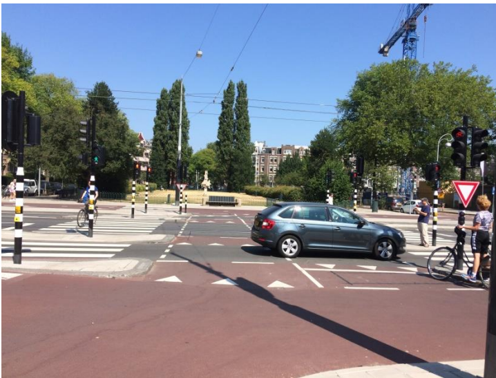
Picture 14: Amsterdam, Valeriusplein, bicycle crossing with curb protection; Source: own picture (June 2018)
