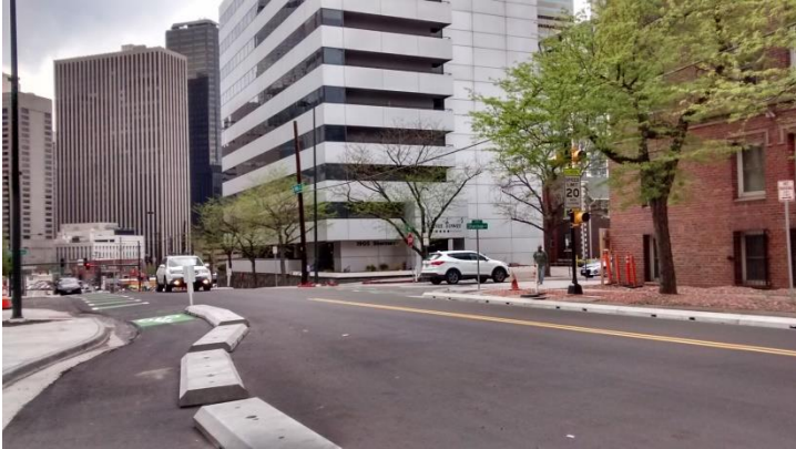
Picture 13: 19th street curb protected bike way; Source: own picture (May 2018)
