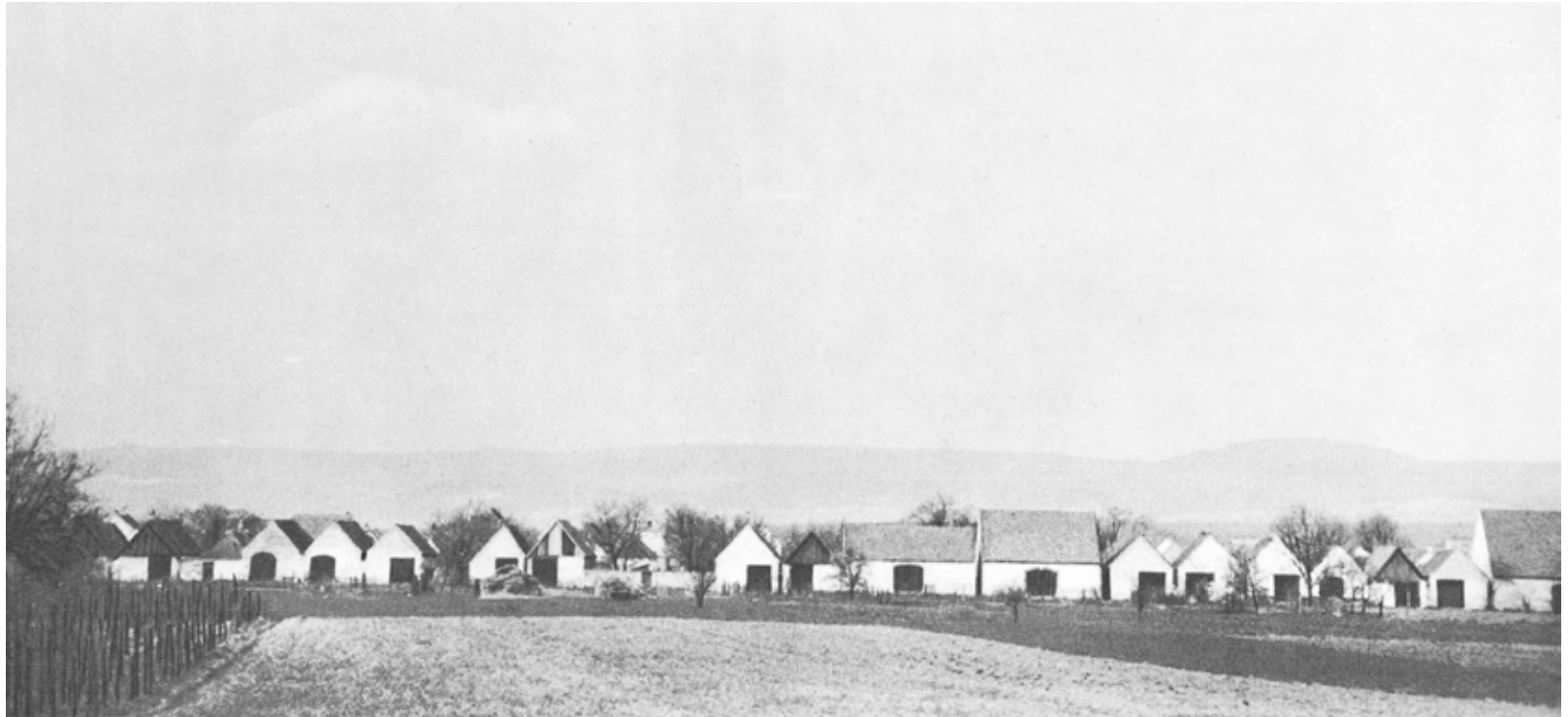
Abb. 11: Häuserfront in Oslip, Nordburgenland
