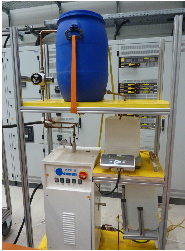
Figure 4.8: Ghidini steam generator (S-2) with construction for adjusting steam mass flow rate
