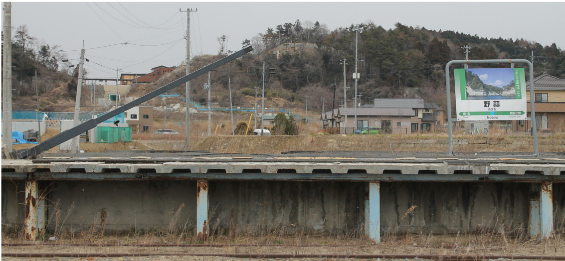
Fig. 4 Abandoned tsunami-damaged railway station and the settlement surrounding it (front), and newly-built station on the hill where the entire settlement was relocated (Source: own photograph taken in March 2014)
