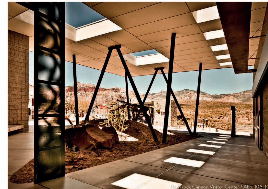
Red Rock Canyon Visitor Center / Abb. 108-109
