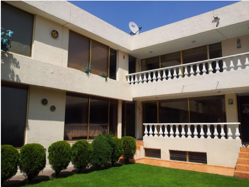
Figure A8. Herradura's residence West and South façades.
