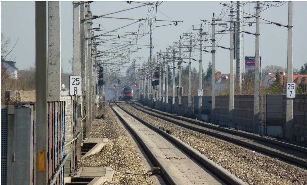
Figure 1.1: Train track with noise barriers
