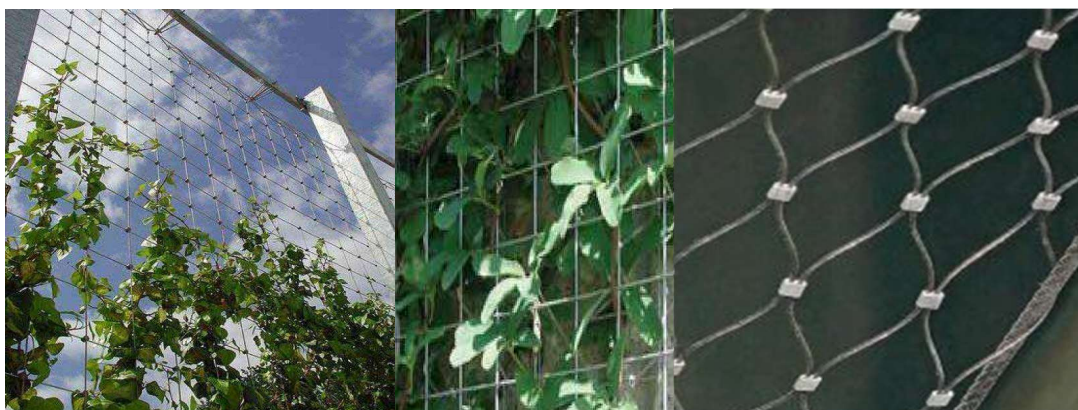
Figure 10 : Steel cables mesh construction (Source: GREENSCREEN 2017 )
