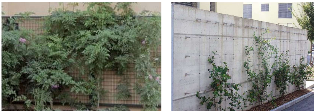
Figure 11 : Steel ropes and trodden rods construction (Source: GREENSCREEN 2017 )
