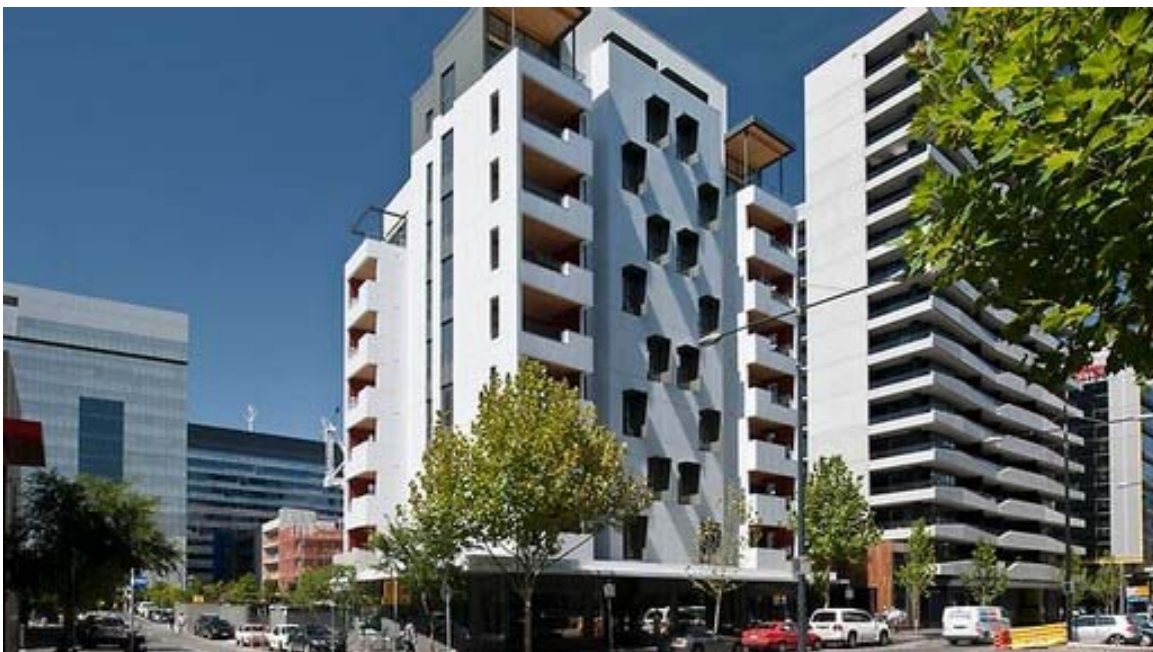
Abbildung 9.26: Forte Living Tower in Melbourne [119]
