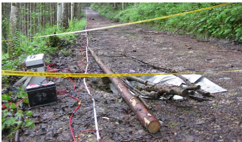
Figure 2: Picture of the provisionally covered entrance of Forststraßeneinbruch, also visible the ERT instrument.
