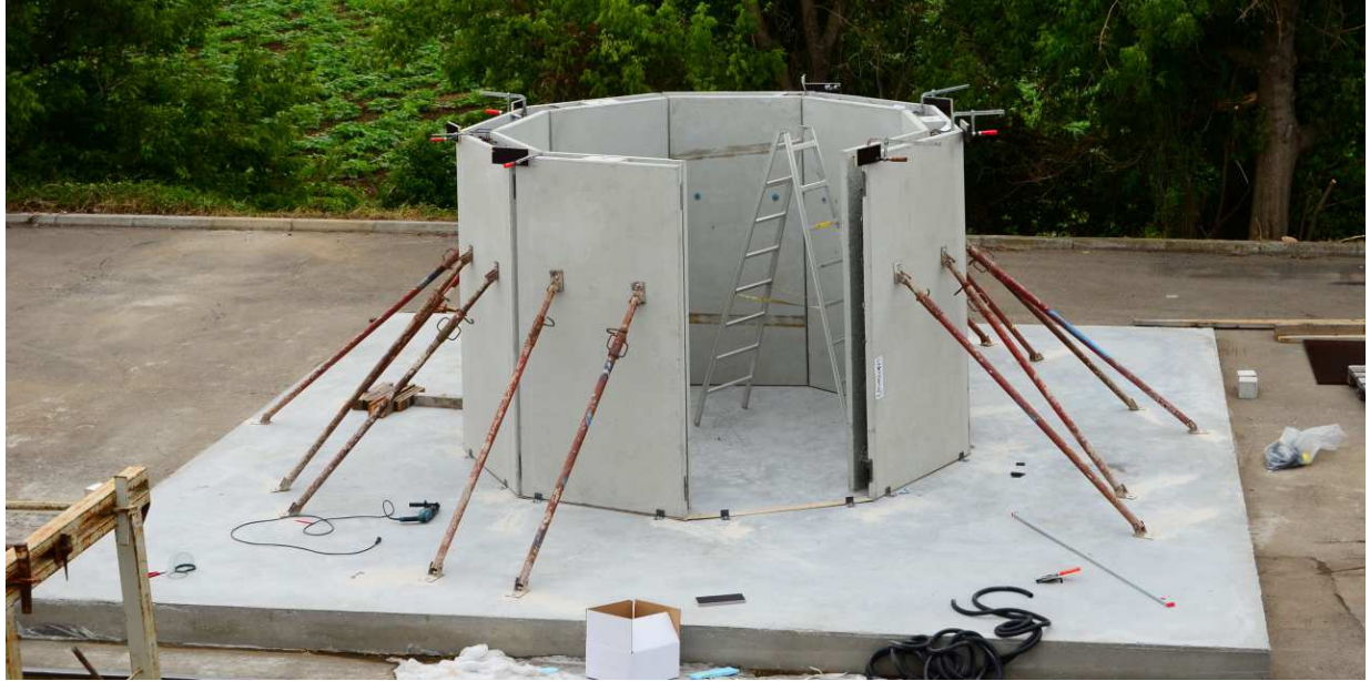
Figure 4.62: Assembled ring segment without the last element
