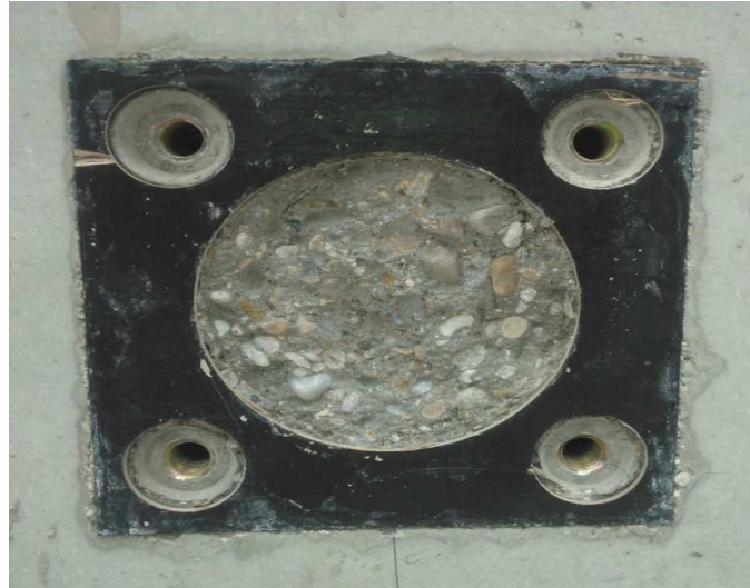
Figure 4.79: Concrete pump opening after concreting
