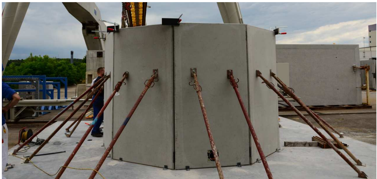
Figure 4.61: Arranged and supported half ring segment- view from outside
