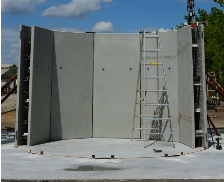
Figure 4.60: Arranged and supported half ring segment- view from inside
