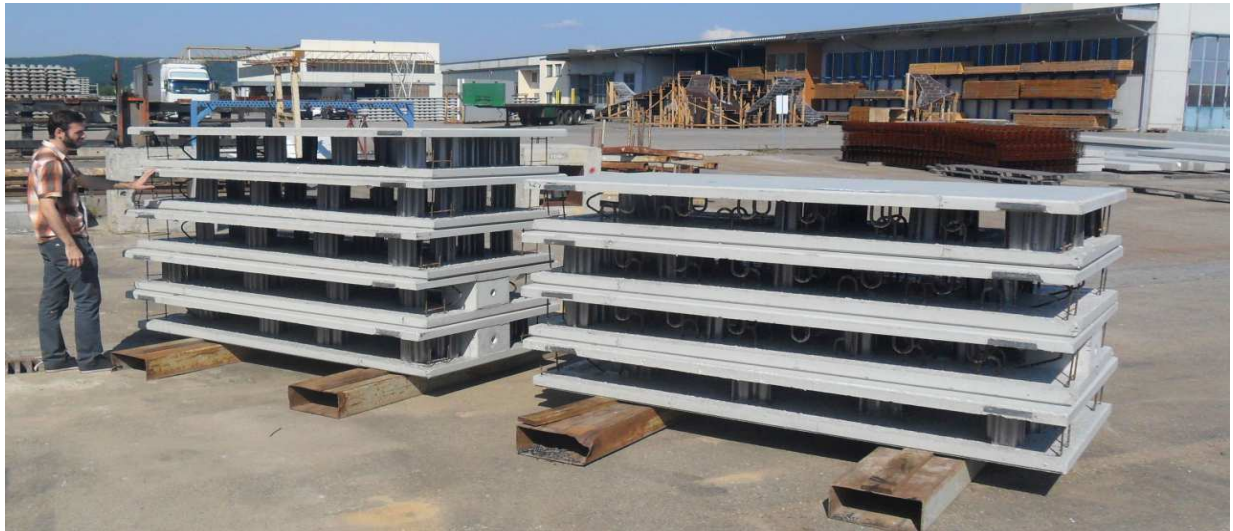
Figure 4.48: All nine double wall elements transported to the building site and ready to be put together to form a mock-up segment
