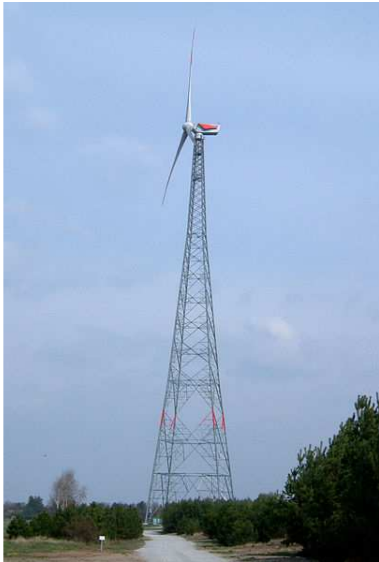
Figure 2.9: Fuhrländer Wind Turbine Laasow in Germany, taken from [14]
