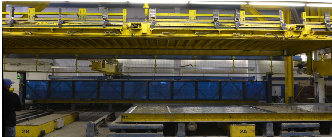
Figure 4.42: Positioning of the pallet with the recent concreted second shells
