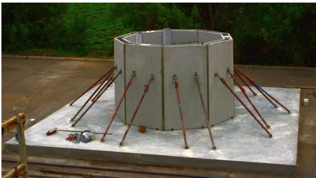
Figure 4.70: Assembled mock-up with bracings
