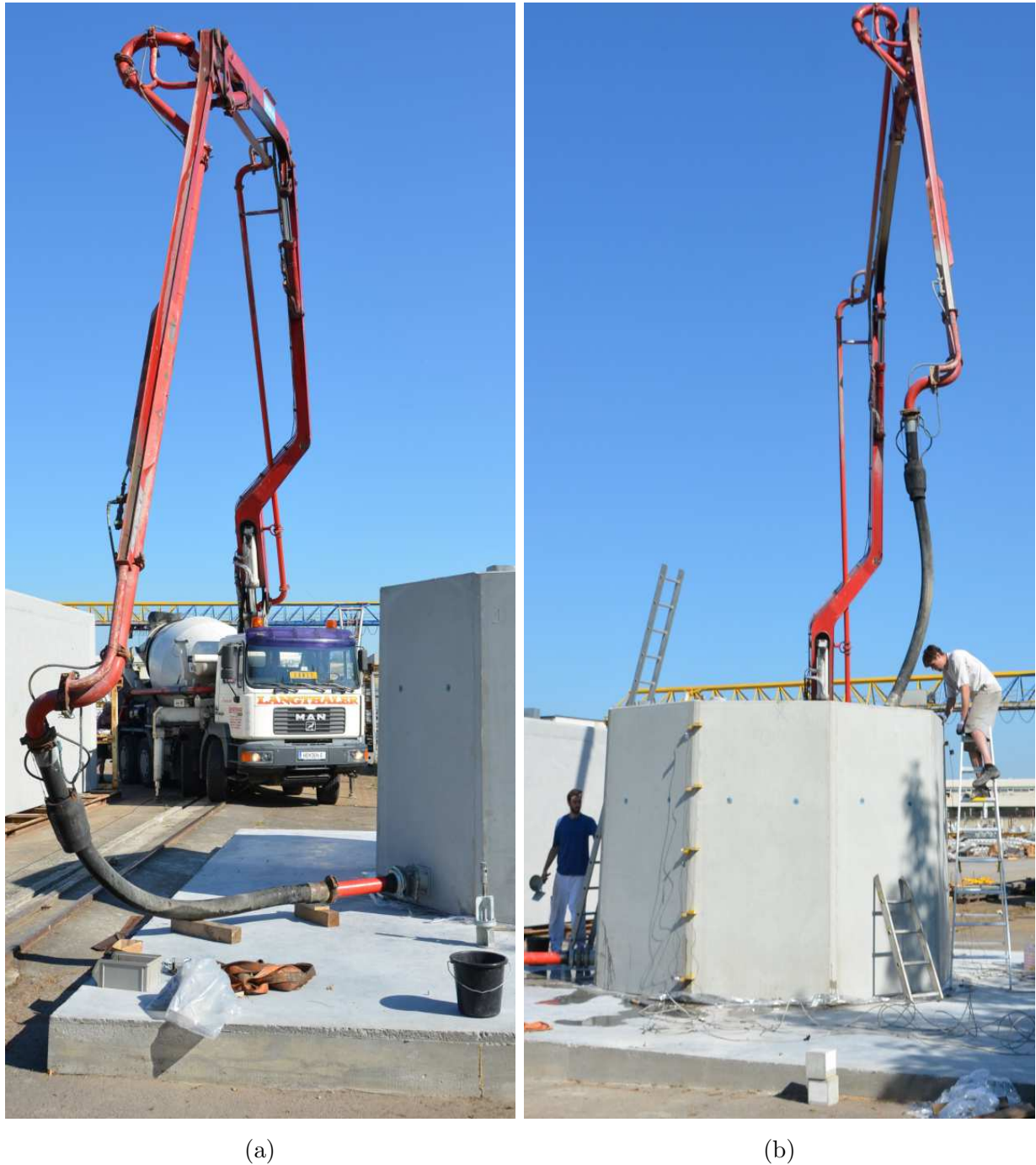
Figure 4.77: Concreting of the mock-up; (a) under pressure from below; and (b) from above
