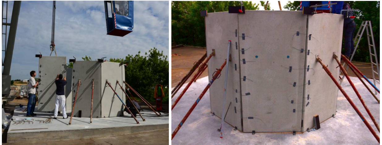
Figure 4.63: Positioning of the last double wall element; (a) positioning of the last element with the crane; and (b) last element at its foreseen position
