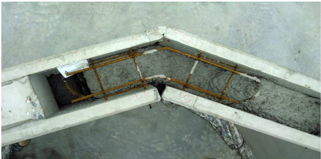
Figure 4.80: Top view of concreted ring segment showing the accessibility of the concrete blocks
