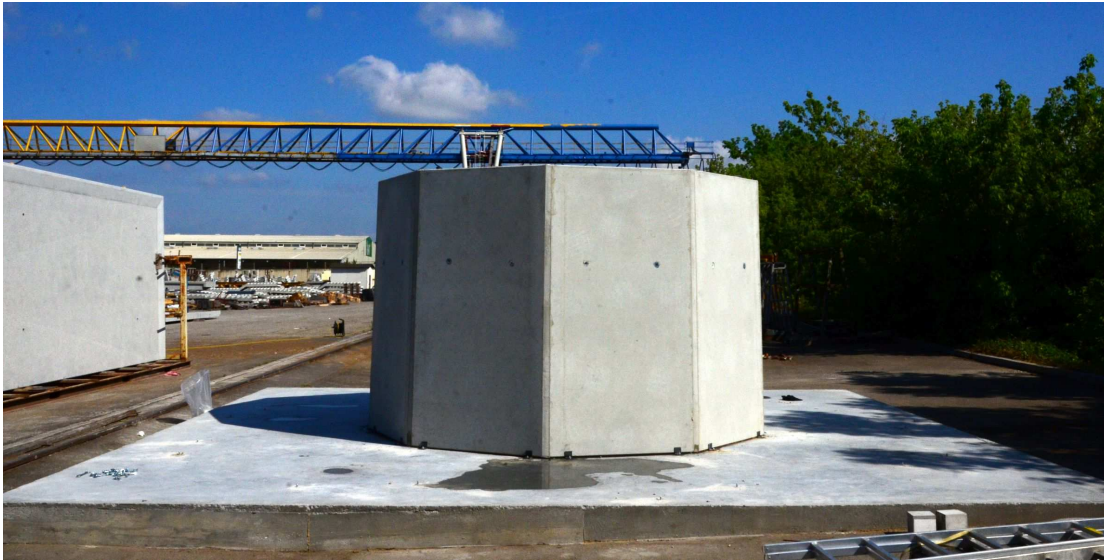
Figure 4.71: Assembled mock-up without bracings
