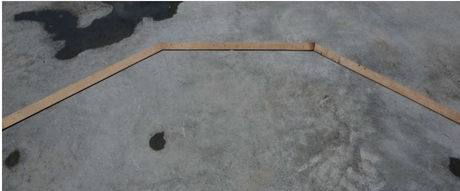
Figure 4.52: Wooden planks for the easier arranging of the elements
