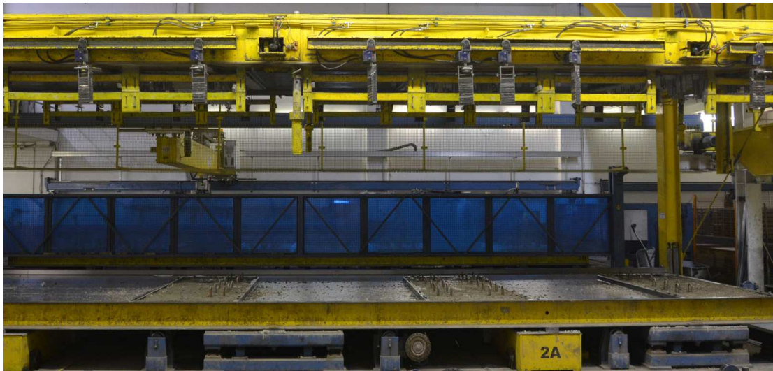
Figure 4.44: Descending of the upper shell into the lower one
