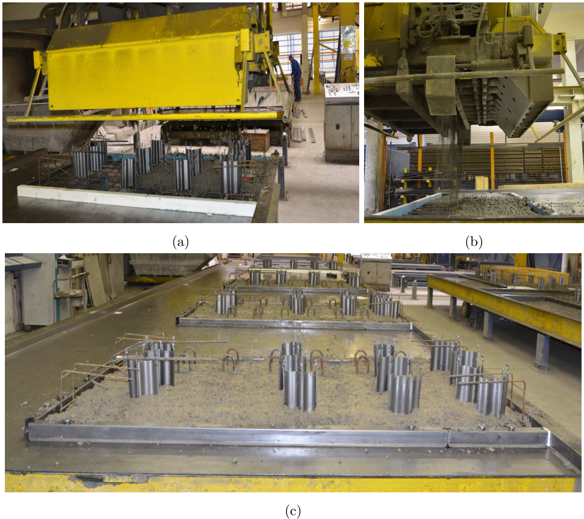
Figure 4.38: Concreting of the elements; (a) side view of the concrete spreader; (b) bottom view of the concrete spreader; and (c) formwork filled with concrete
