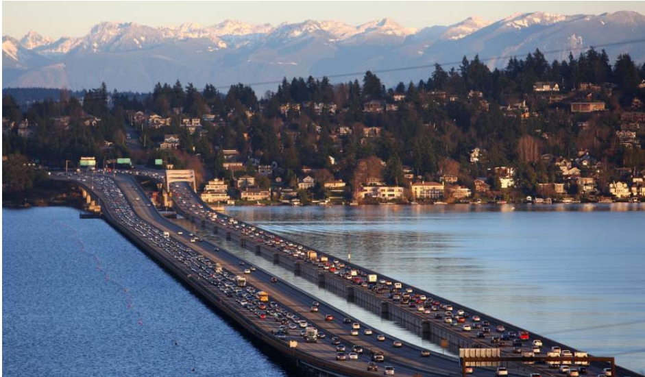
Abbildung 2-2: Lake V. Murrow Floating Bridge (Gutierrez, 2012)
