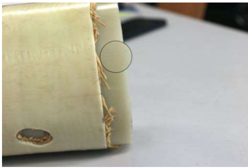
Figure 1.7: End of pipe 1
