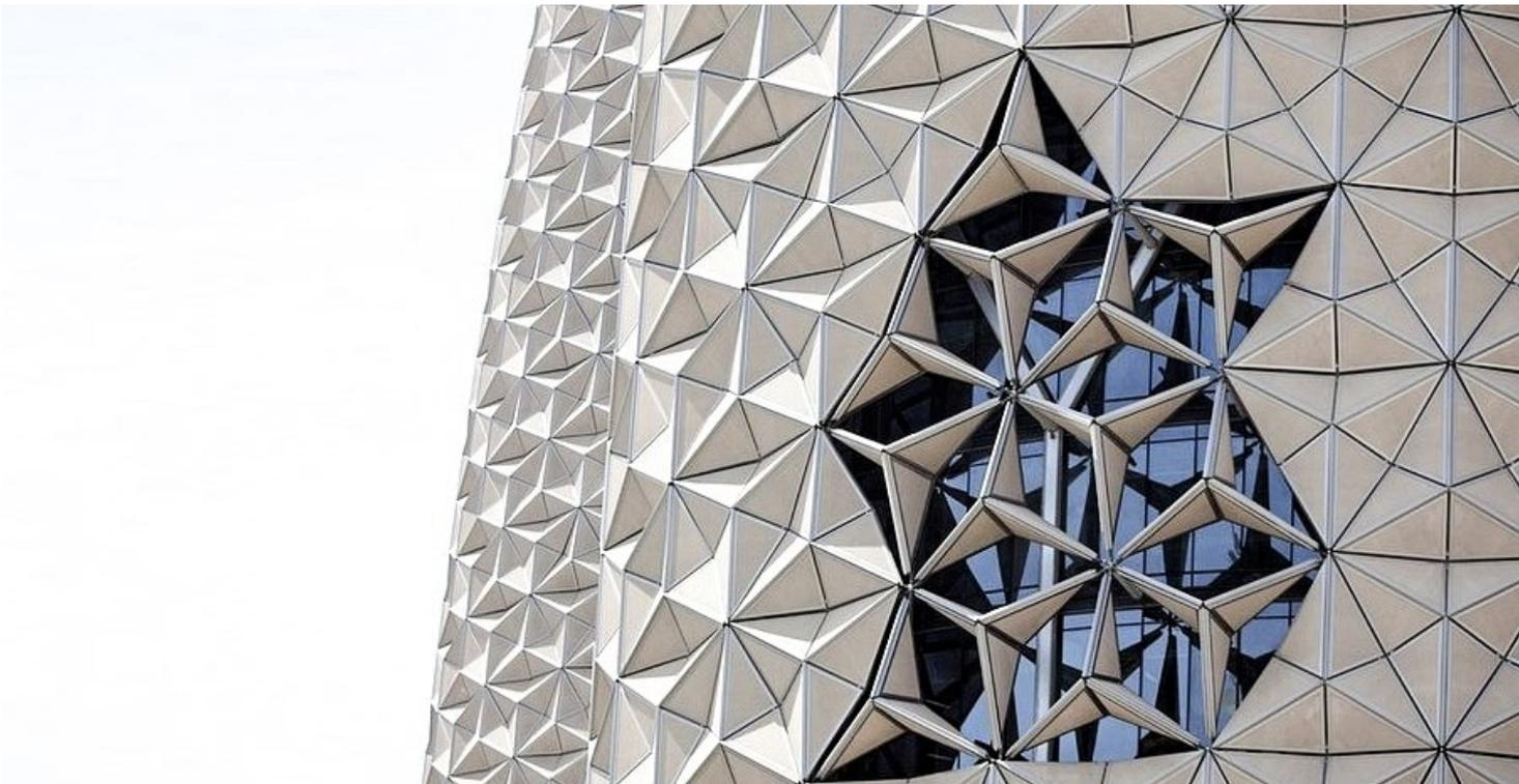
photo M15 **"rigid body structure"**, responsive facade Al Bahar Towers, Aedas Architects 2012
