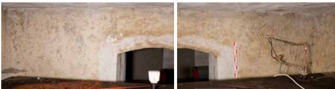
Wand West Wand West
