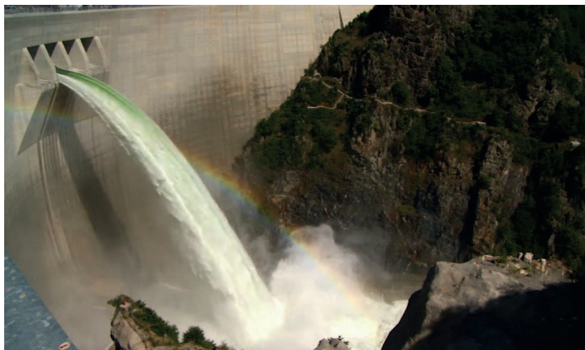
Figure 1.2: Tsankov Kamak (Bulgaria): spillway test. Courtesy of D. Kischlat (2010)
