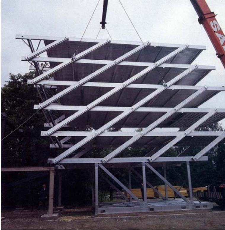
Figure 4.9 The prototype during the erection process in Germany.
