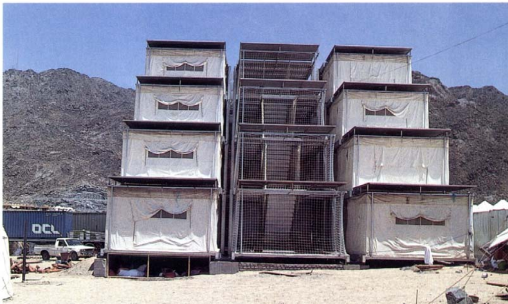
Figure 4.13 The foldable structure fitted with the canvas to form all the accommodation chambers and other utilities. In the centre of the unit can be seen the vertical circulation cluster which can also be used for storage, 1985.
