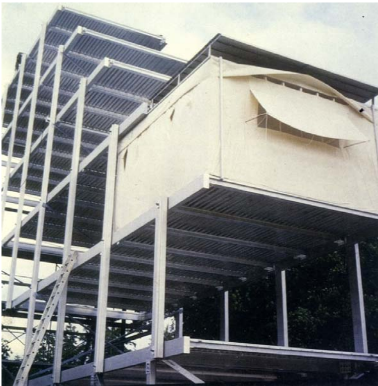
Figure 4.10 The prototype in Germany being fitted with the living module canvas.
