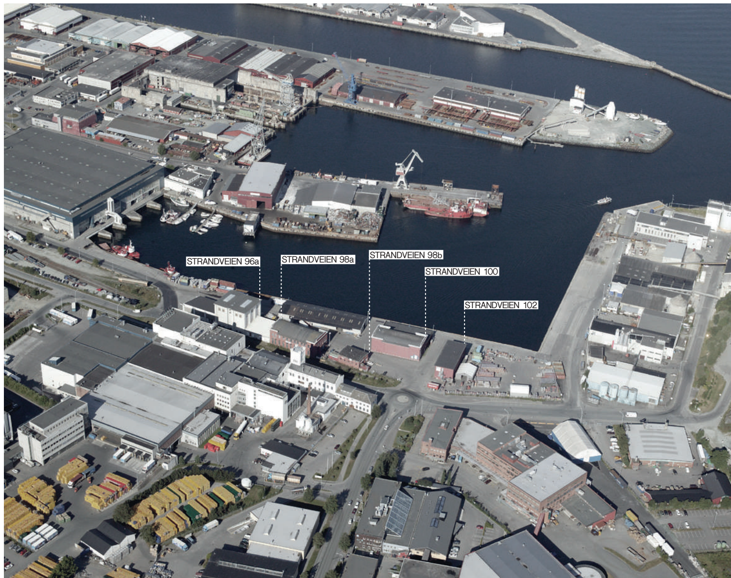
Fig.27 Project site at Nyhavna east with existing buildings on site;
