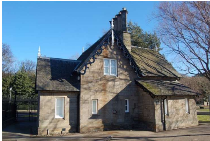
Fig. 57 View of Holyrood Park Lodge (Historic Building Energy Retrofit Atlas, 2019)
