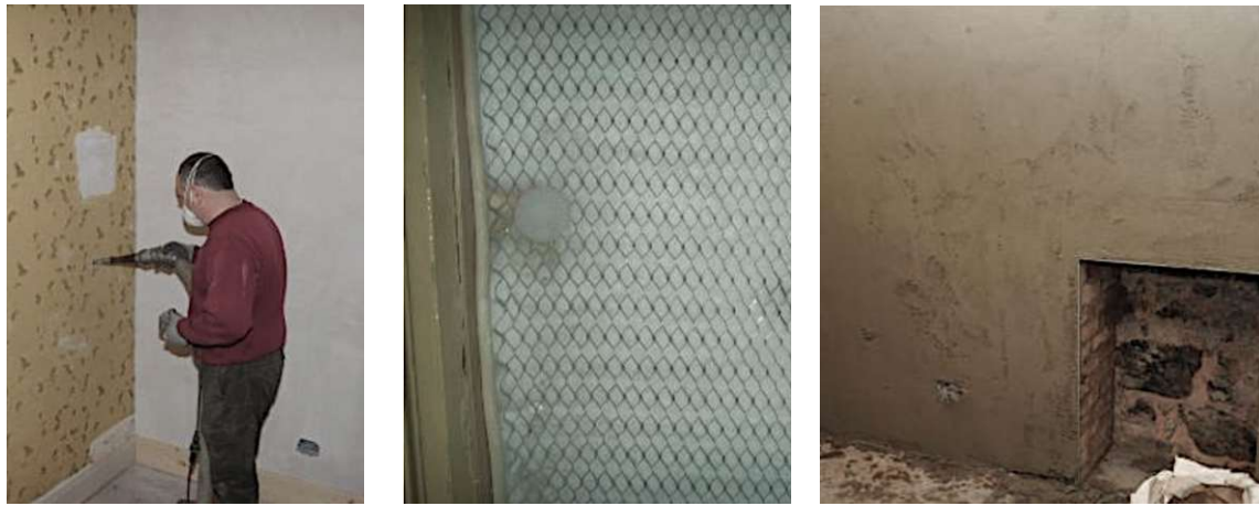
Fig. 53 Left: Blowing in the cellulose fiber, right: Aerogel blanket held behind mesh, right: First coat of plaster on top of the mesh/insulation layer (Historic Scotland, 2012, 13-14)
