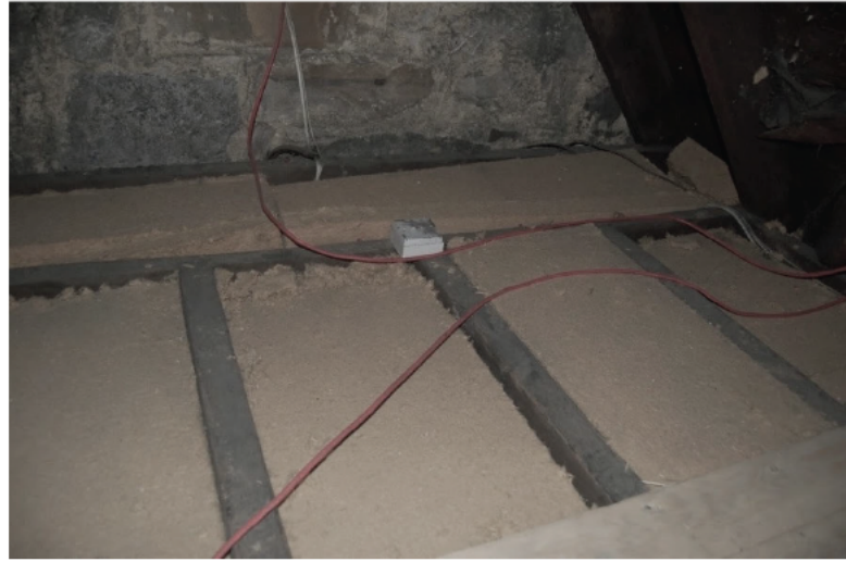
Fig. 60 Left: The warm roof with wood fiber between the rafters, right: The cold roof with wood fiber insulation between the rafters (Historic Building Energy Retrofit Atlas, 2019)
