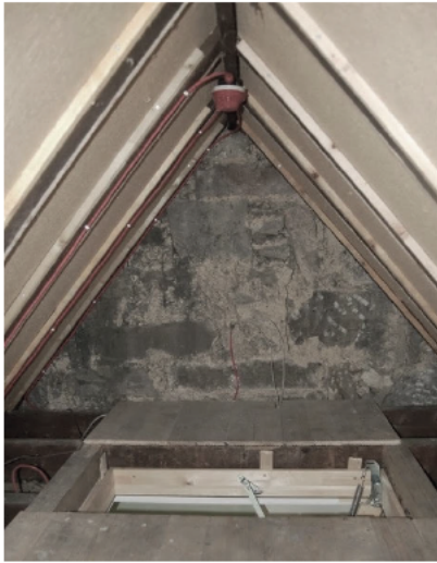
Fig. 60 Left: The warm roof with wood fiber between the rafters, right: The cold roof with wood fiber insulation between the rafters (Historic Building Energy Retrofit Atlas, 2019)
