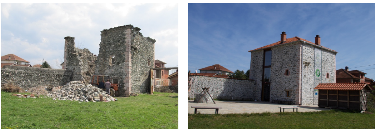
Fig. 36 Reconstruction and adaptive reuse of the Kulla Ruste Zeqiri, Junik as a Regional Tourism Center, during 2001-2002, Left: Kulla before (CHwB Kosova, 2001), right: Kulla after intervention (CHwB Kosova, 2016)
