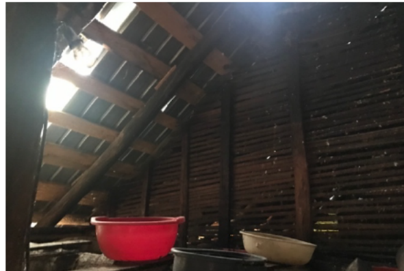
Fig. 209 Left: Damp in the ceiling of a used bedroom, 2021, right: Holes in the roof and baskets for water, 2021
