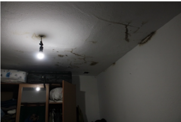
Fig. 209 Left: Damp in the ceiling of a used bedroom, 2021, right: Holes in the roof and baskets for water, 2021
