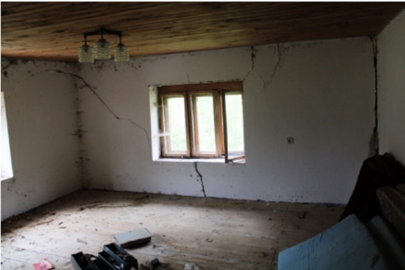
Fig. 208 Left: Constructive cracks in the abandoned part, 2021, right: Damaged plaster and window, 2021
