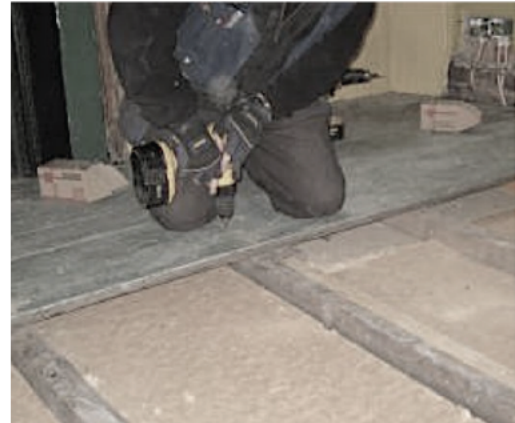
Fig. 52 Left: Detail of the floor insulation, right: Floor being fixed down over wood fibre bats (Historic Scotland, 2012, p.10-11)
