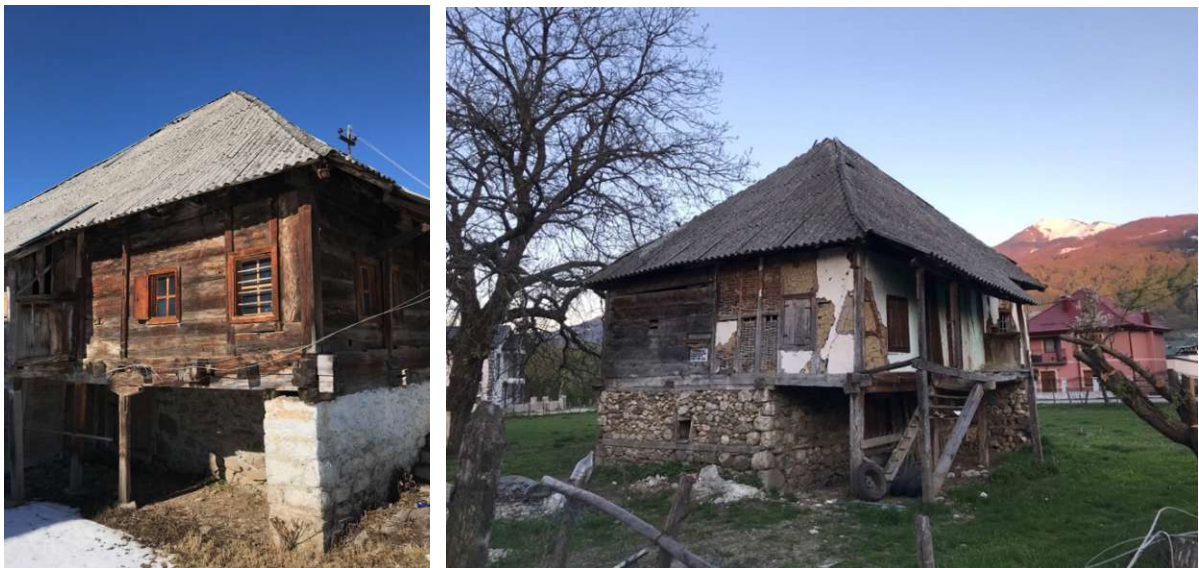
Fig. 9 Left and right: Houses with stone ground floor and timber upper floor (Labeatët, 2021)
