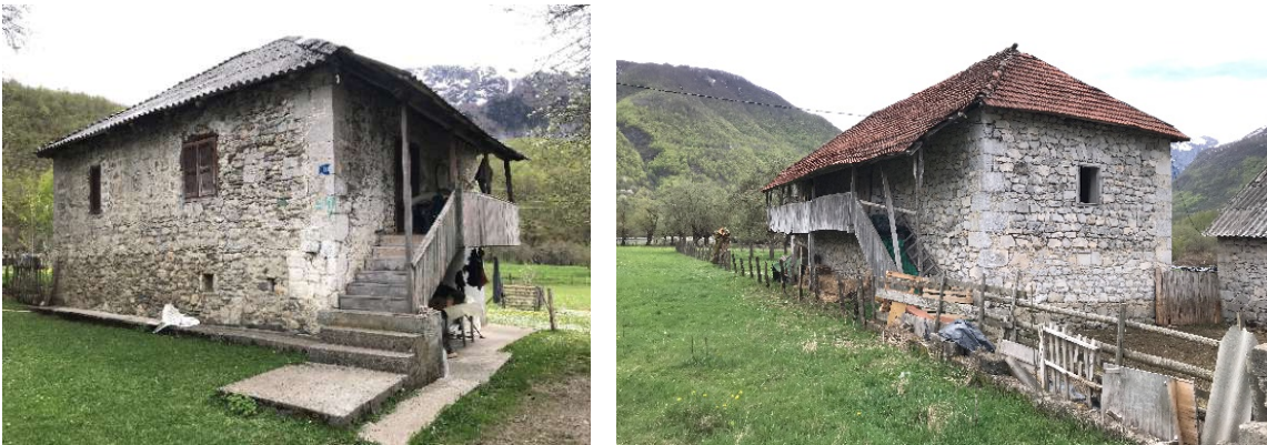
Fig. 10 Left and right: Stone houses in Vuthaj (Labeatët, 2021)
