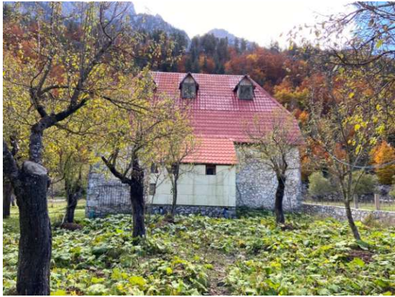
Fig. 195 Left: New annex added in the north facade, 2021, right: Rising damp in the west facade, 2021
