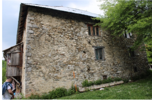
Fig. 207 Left: The damaged roof cover of the building, 2021, right: Cement mortar and enlarged windows, 2021
