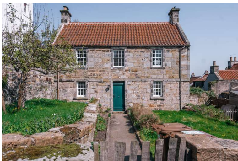
Fig. 55 View of the Wee Causeway cottage (Wanderintwo, 2022)
