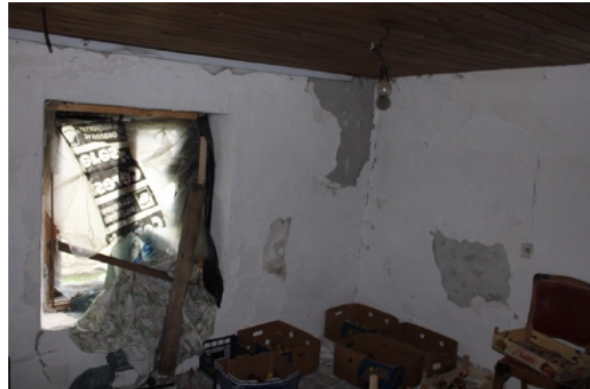
Fig. 208 Left: Constructive cracks in the abandoned part, 2021, right: Damaged plaster and window, 2021
