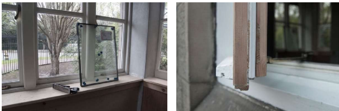
Fig. 59 Left: One of the double-glazed units before installation, right: Draught strips added to casements (Historic Building Energy Retrofit Atlas, 2019)
