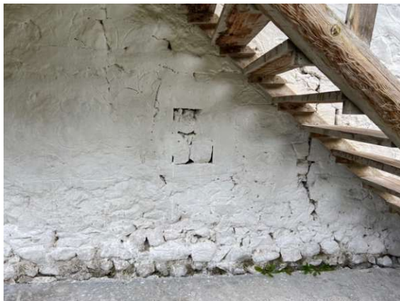
Fig. 196 Left: A closed opening and a crack in south facade, 2021, right: Cement mortar and new windows, 2021
