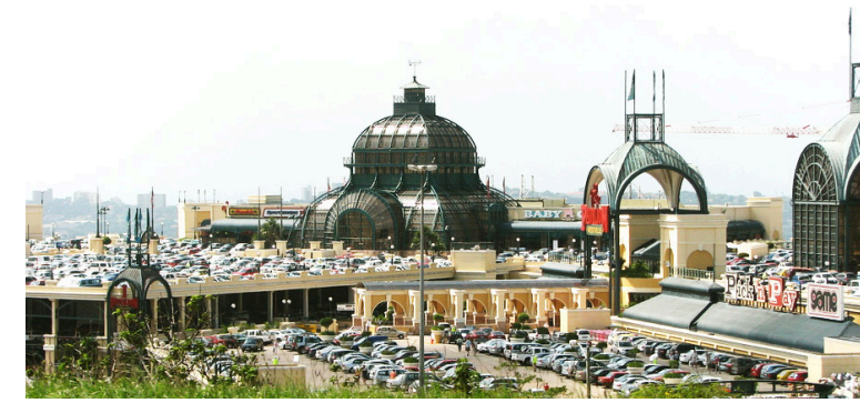
Fig.6 The Pavilion shopping centre in Westville Durban
