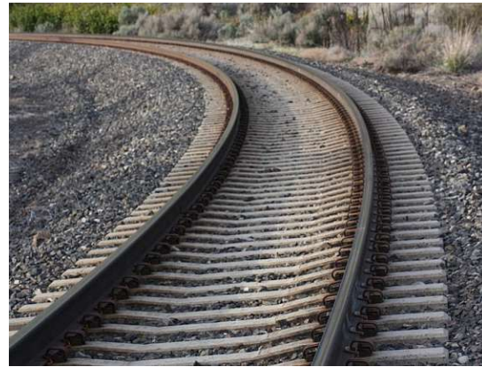
(b) Concrete sleepers
