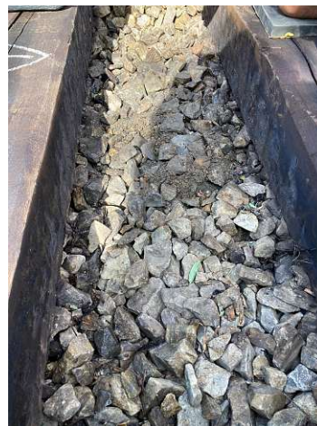
(b) Sleeper bay, bottom edge of the sleeper
