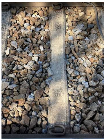
(a) Sleeper bay surface
