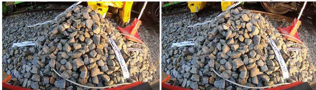
(c) Tamping unit approaching
