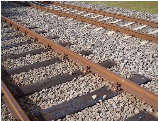
(a) Wooden sleepers
