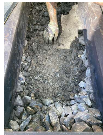
(c) Sleeper bay, upper edge of the subgrade
