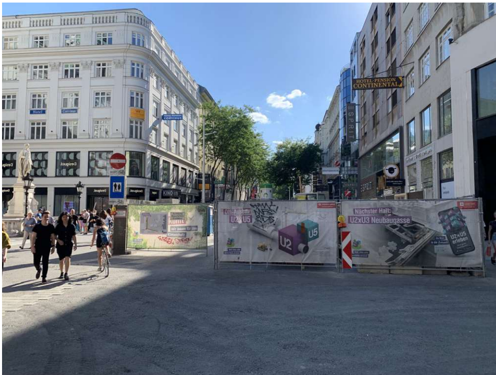
Figure 4.9: Photo of Mariahilferstraße case study. Explanation of the works can be seen on the fences.
