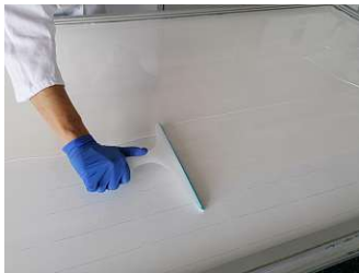
(a) Picture of distributing the Remsolar cover coating.
