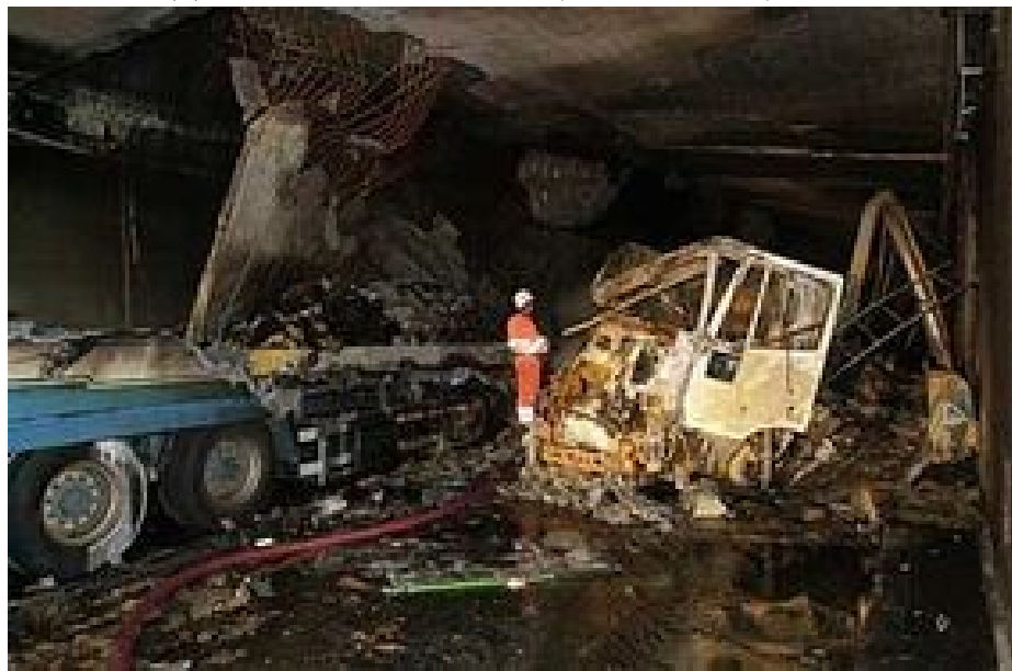
(b) Partially collapsed ceiling and burned out truck (picture by Ti Press)
