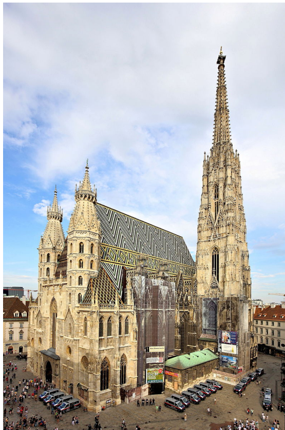
Figure 2.2: St. Stephen's Cathedral is an example of a highly salient landmark. It stands out from its surroundings by its size and noticeably different and rich gothic architecture [Bwa].
