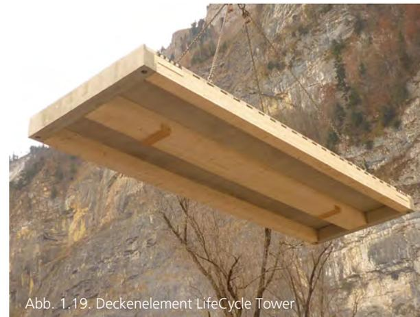
Abb. 1.19. Deckenelement LifeCycle Tower
