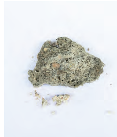
Probe 3, Lager IV, Innenwand
