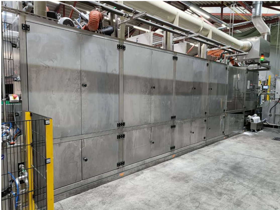
Figure 6.1: Company B - Industrial washing machine for aluminum surface cleaning.
