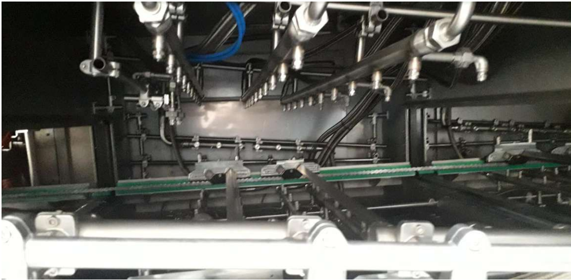
Figure 6.3: Company B - Spraying nozzles and the transport system in chamber one.
