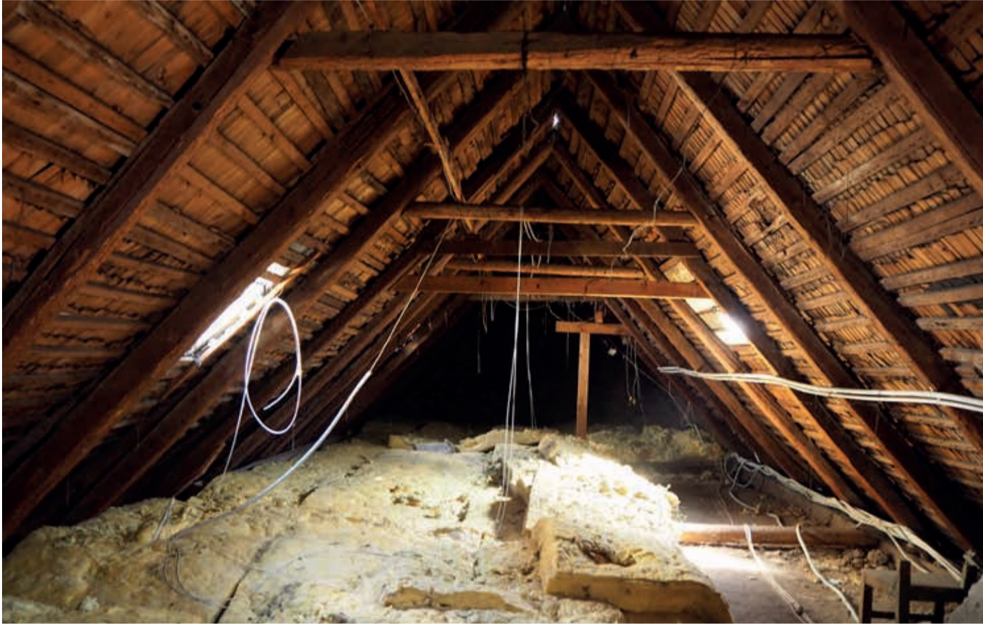
Abb.144 Blick a | Satteldach | Raum 23
