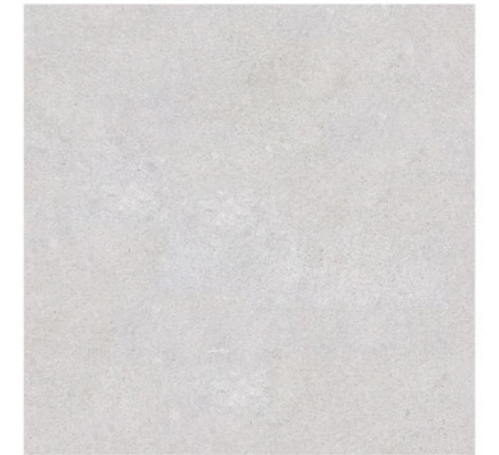
Abb. 90: Decke: Beton (Planschalung, Grauzement)
