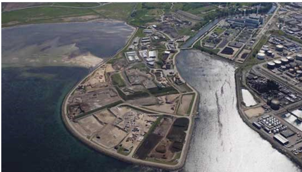
Figure 13 Sysav Waste Site
