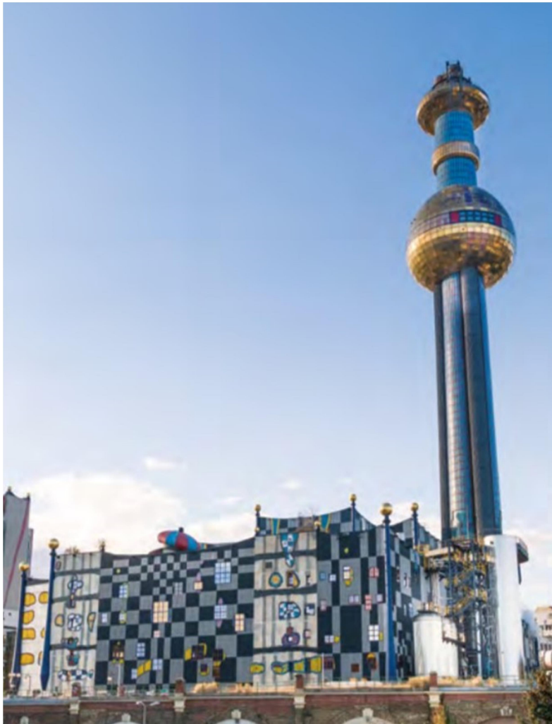
Figure 12 Thermal waste incineration plant Spittelau, Vienna, Austria
