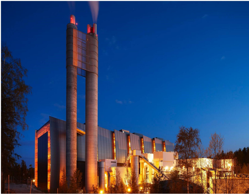
Figure 19 Klemetsrud, Oslo Waste to Energy Plant
