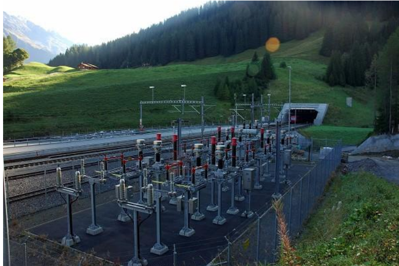
Figure 3.6: Vereina tunnel east portal [35].
