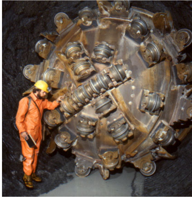
Figure 3.9: Hemerwald tunnel TBM [courtesy, Ewald Tentschert].
