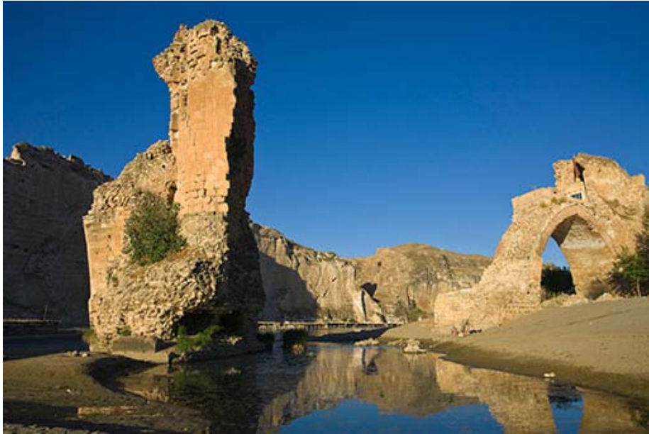
Figure 10 Broken arches and pylons of Eski Koprusu (Source Smithsonian Magazine)
