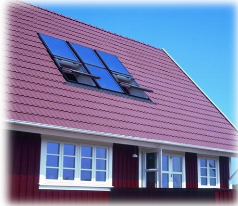
Figure 3.2.3.4: Roof Integrated Flat-Plate Collectors – Residential Building in Denmark Source: Renewable Heating & Cooling, European Technology Platform
