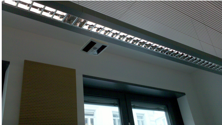
Figure 50. Occupancy detection based on a wireless motion sensor
