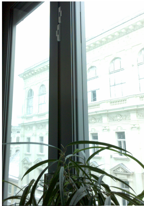
Figure 51. Contact sensor used to measure window state
