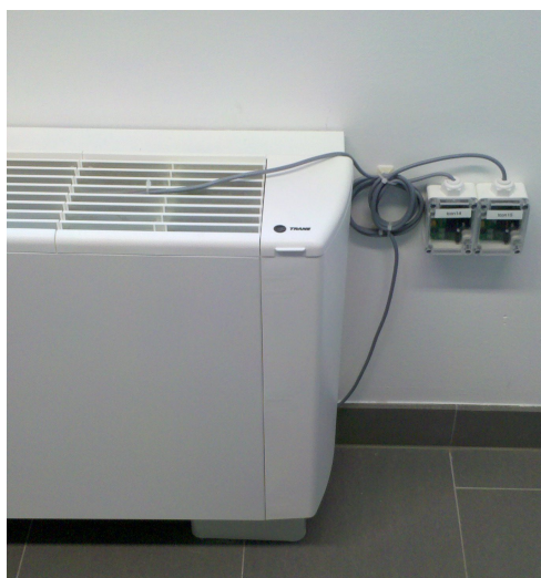
Figure 48. Sensor setup at the fan-coils
