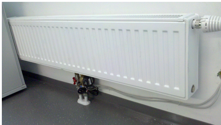
Figure 47. Heat meters installed at radiators
