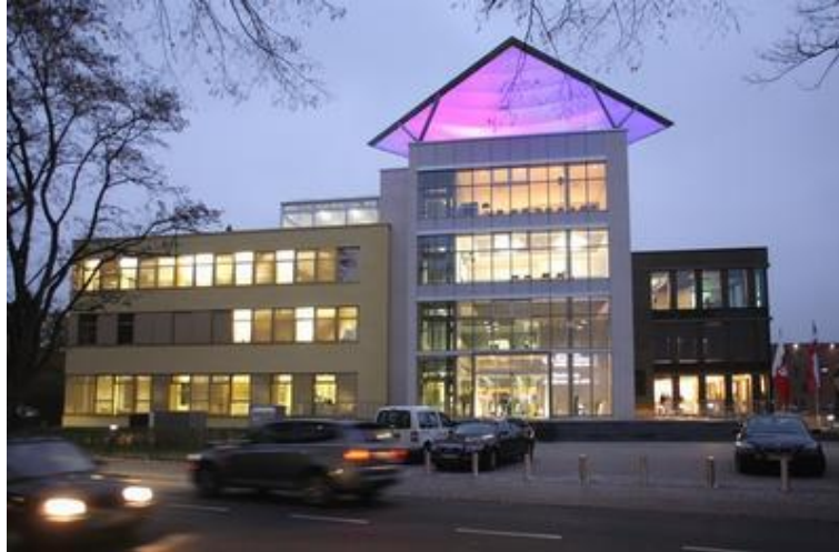
Figure 1.13: inHaus 2 – Smart Building [34]
