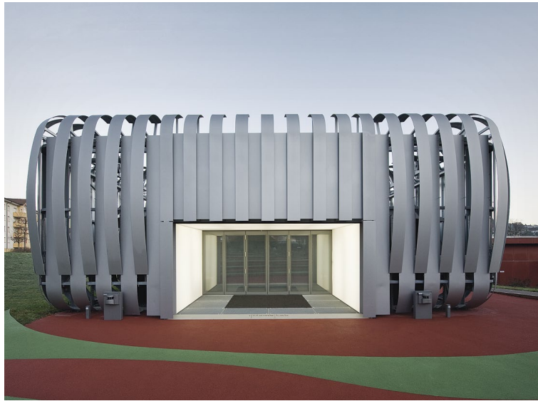
Figure 1.14: iHomeLab exterior view [37]
