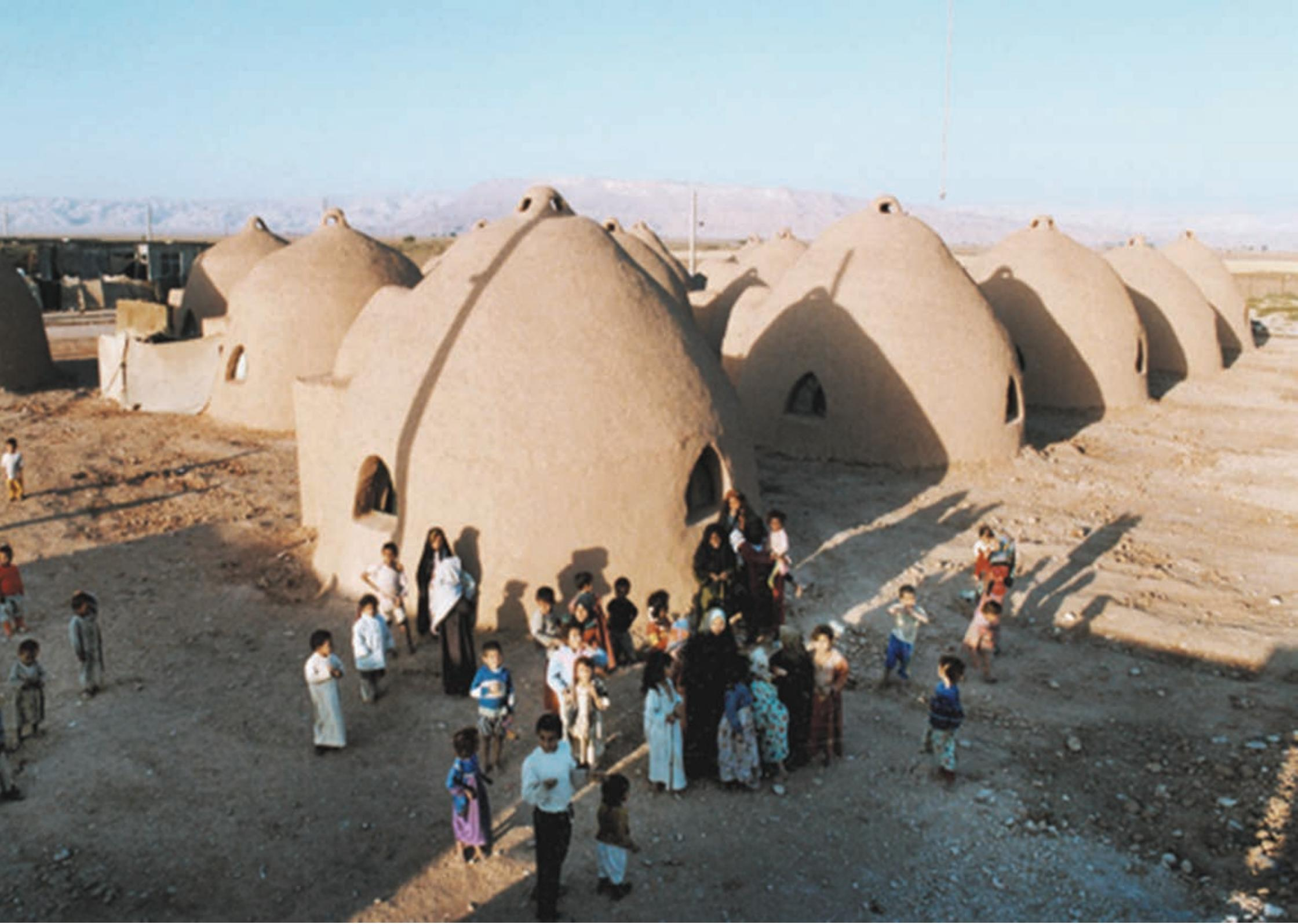
Superadobe is a form of earth bag construction that was developed by Iranian architect Nader Khalili<sup>8</sup>. The technique uses layered long fabric tubes or bags filled with adobe<sup>9</sup> to form a compression structure. The resulting beehive shaped structures employ corbelled arches, corbelled domes, and vaults to create single and double-curved shells that are strong and aesthetically pleasing.
