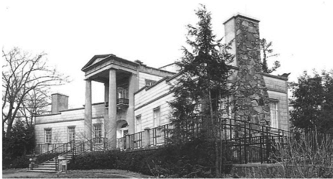
Abbildung 44: Burrit Mansion House, Huntsville, Alabama, USA, 1938
