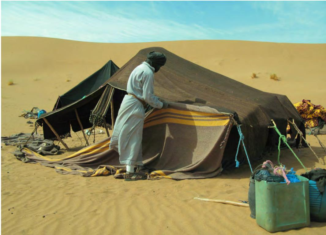
*image 3.049: Tuareg elder of the Nouaji tribe connecting the wall blanket with metal pins to the tent roof; Sahara (Zagora region) 2008*
