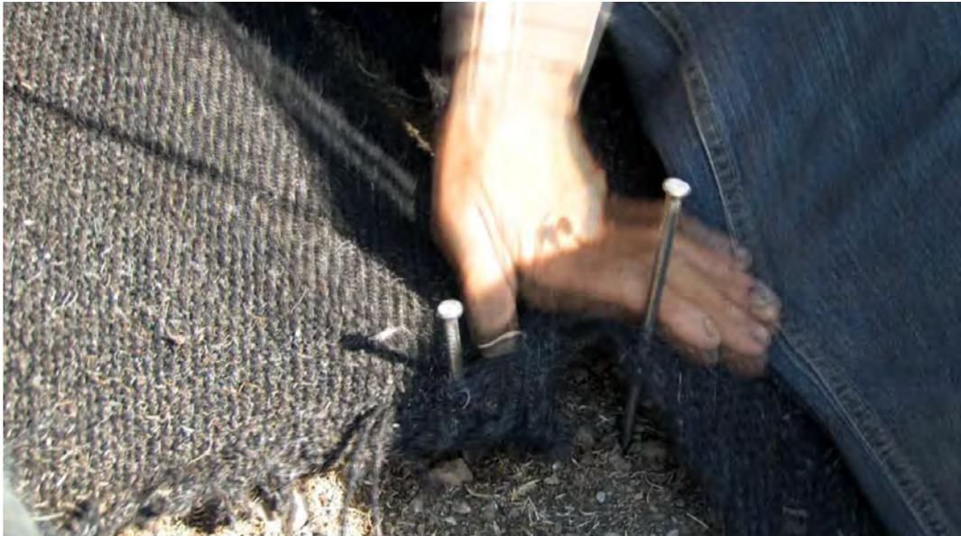
*image 4.024: Abutted seam step 3. Pulling the edges together.*
