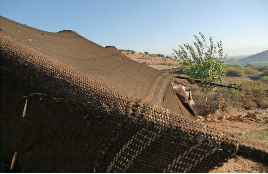
*image 3.012: Yörük tent with siyek kolanı (see element “d” on the sketch after Eröz). A wooden pin (sitol çöpü or çivi) is shown left below.*
