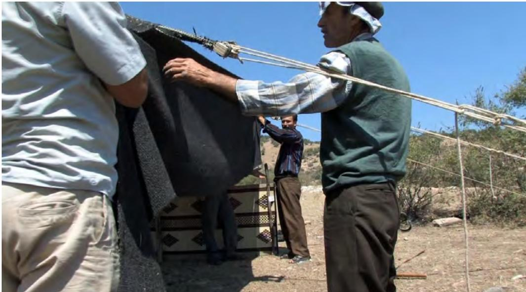
*image 4.049: The length for the wall panels is measured. Afterwards, two panels for each side will be stitched together without any pre-stretching.*
