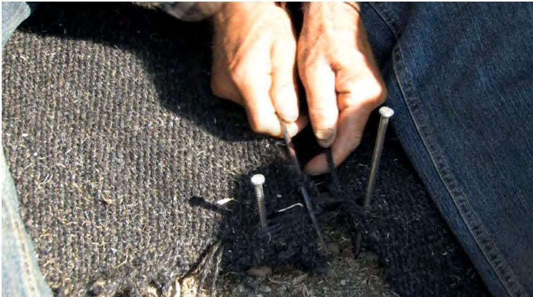
*image 4.025: Abutted seam step 4. Now, the other side is stitched from underneath. All stitches must be started underneath. As seen in these pictures, “bent narrow twists” were used as needles.*
