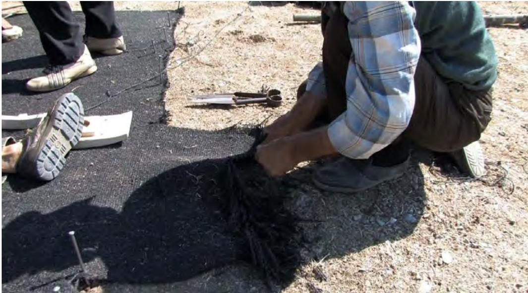
*image 4.032: The flags of the centre panels can be frizzled if desired. The frizzled ends cover the ridge hole lightly, keeping off flies and allowing ventilation.*
