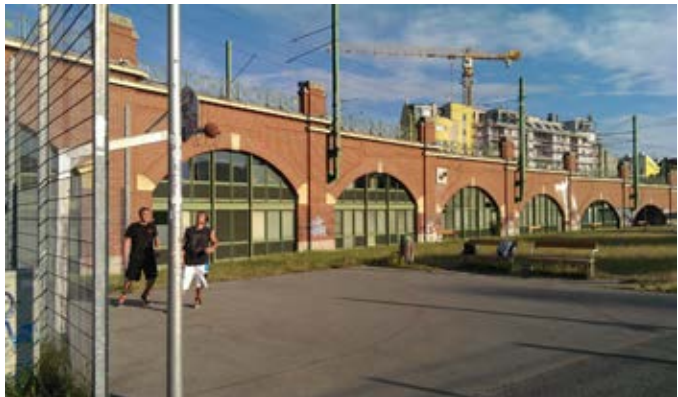
Abb. 43 Trendsportanlage U4/U6 Linse - Basketball
