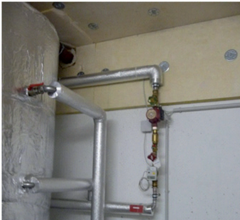
Fig.29 4cm insulation at hot water room
