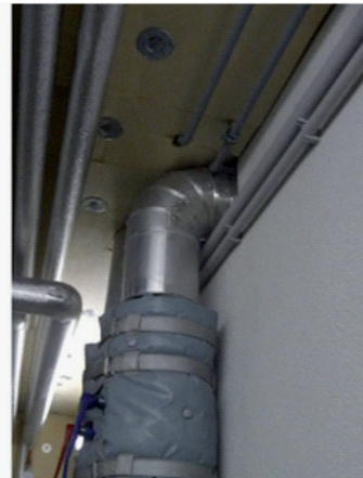
Fig.30 4cm insulation at hot water room
