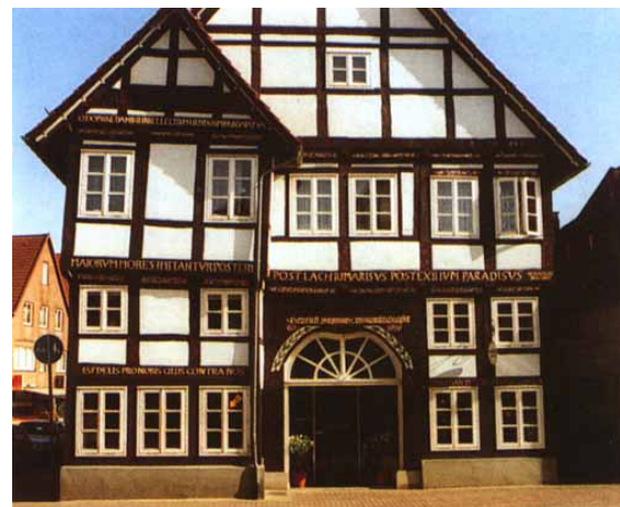
Fig 3.1.e – Timber frame house; Springe, Germany
