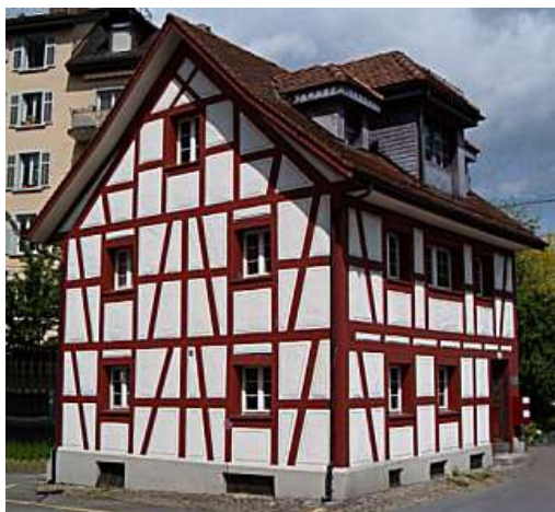
Fig 3.1.d – Timber frame house; Lucerne, Switzerland
