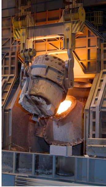
Figure 8.1: AOD converter (Source: Siemens VAI)
