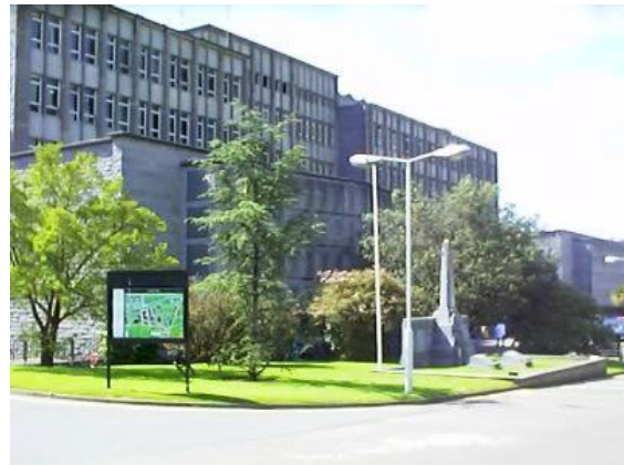
Fig. 3.4.2. Kane building with anemometer placed on the rooftop.
