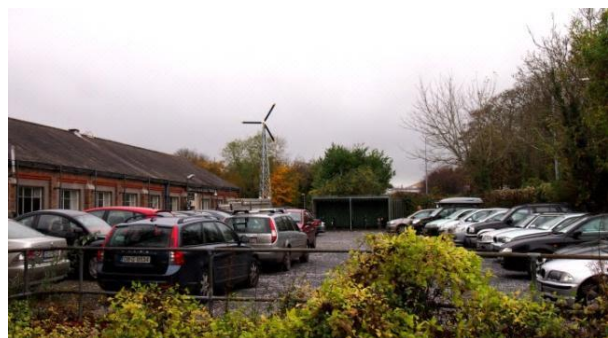
Fig 4.1.1. Bergey Excel 10 turbine on UCC Campus, looking east.
