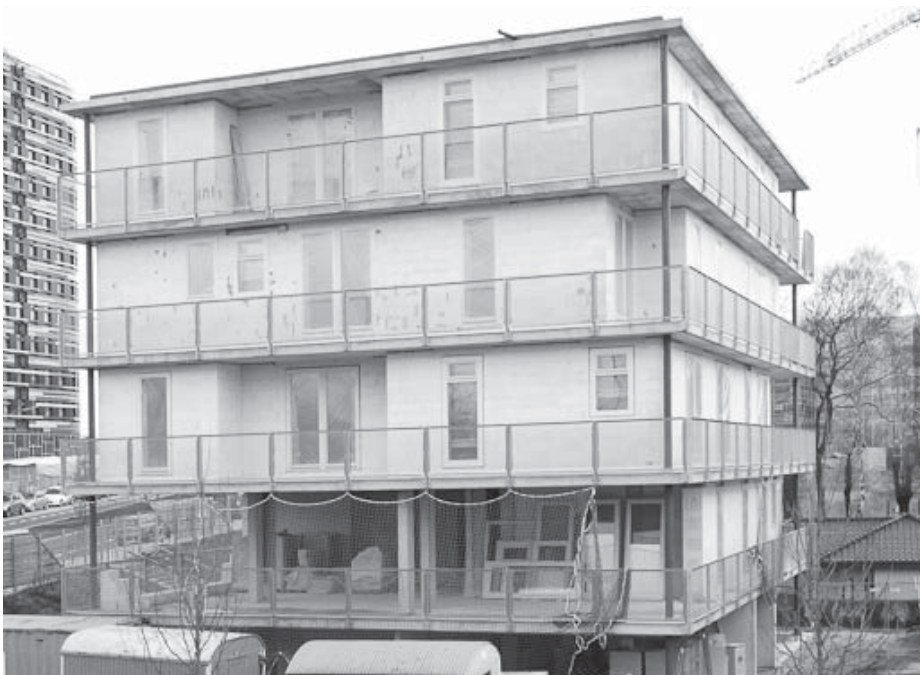
Fig. IV.4.1 Shelf Housing under construction, February 2013. Source IBA-Kunz
