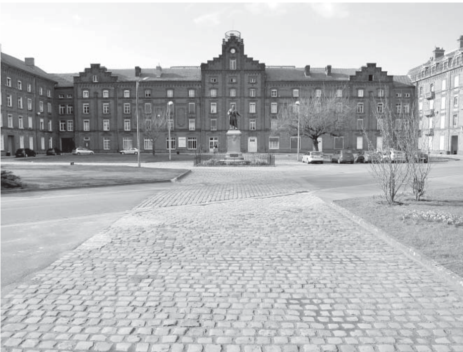
Fig. IV.3.1 View of the central pavilion from the access courtyard
