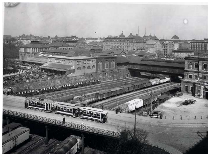
Fig. 42 Great Market Hall, 1928. View of the market halls, in the foreground the Ungar Bridge with a view of the tracks of the connecting railroad and the city railroad. ©MA8 Wiener Stadt- und Landesarchiv
