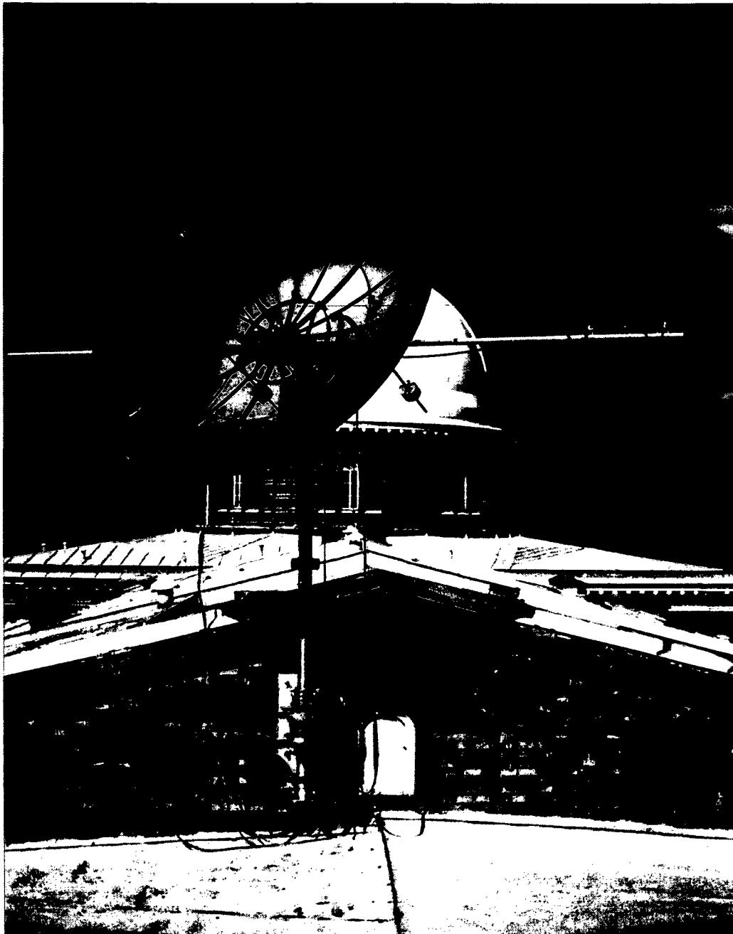
Figure 2.14: Vienna ground station antenna structure. The structure consists of a main rod and a rotating rod. On the upper left the receive antenna, a parabolic dish with a diameter of 3 m can be seen. On the upper right is the transmit antenna, a Yagi antenna group consisting of four single Yagi antennas. Also the rotators for azimuth and elevation can be seen.
