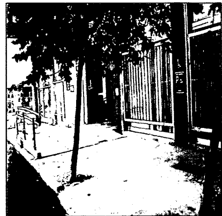
Fig. 16-12: A rare sight: a PwD's parking lot kerow free and a ramp with railing and smooth inclination
