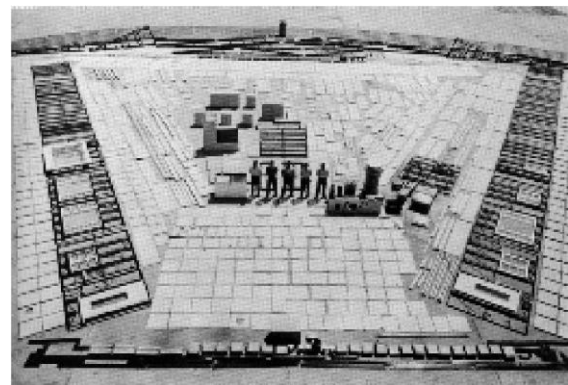
Figure 2.6. Building components of the Lustron-house, Albany, New York (Westra J.1990)
