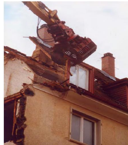
Figure 2.9. Sorting with grippers (Rentz, Seemann, Raess, Schultmann,2003)
